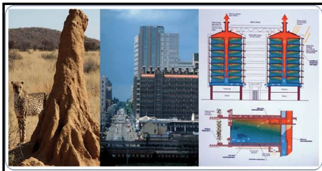
Figure 3: Showing the Pearce Eastgate Project Inspired from Termite Mounds That Have the Ability to Produce Natural Heating and Cooling
