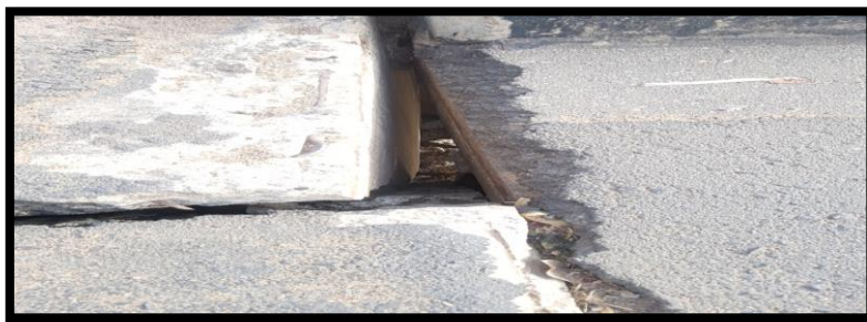
Figure 4: Image Showing Abutment Movement from Bridge Deck
