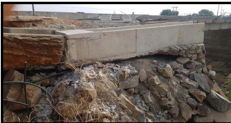
Figure 5: Image Showing Boulders Dump against Abutment
