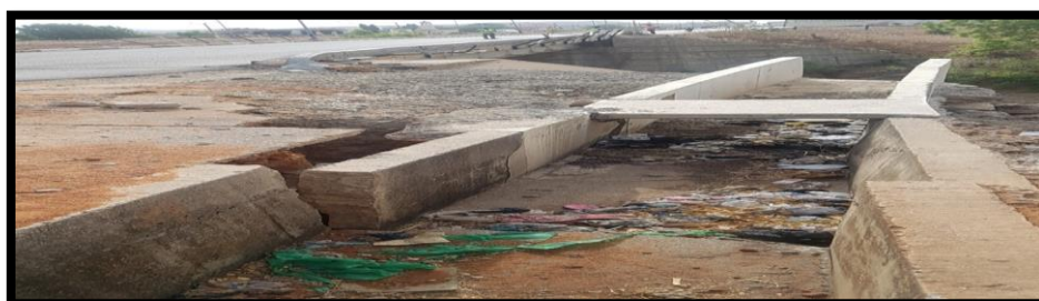
Figure 3: Image Showing Drainage Effect against the Abutment
