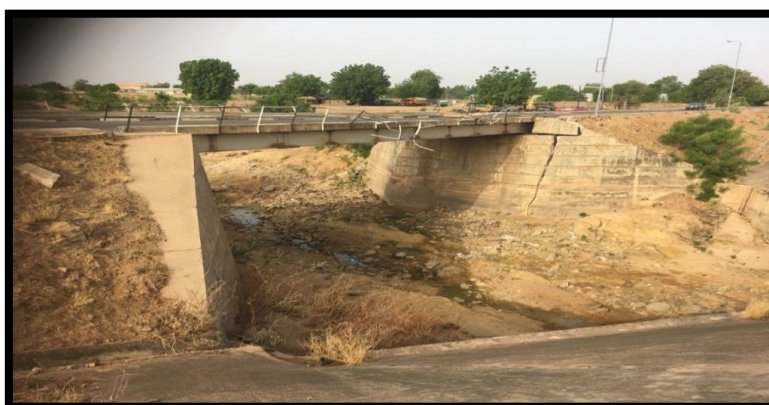
Figure 2: Image Showing Tilted Abutment
