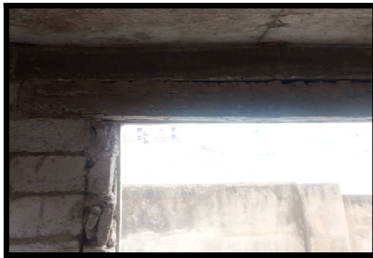
Figure 5: Sagging at Window Opening
